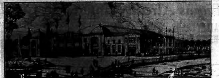
Construction has begun on the Casino at Rye Beach, planned by the County Park Commission to supplement Playland. When completed, it will have one of the largest year-around recreational centers in the country, and will provide a large amount of winter recreation.
